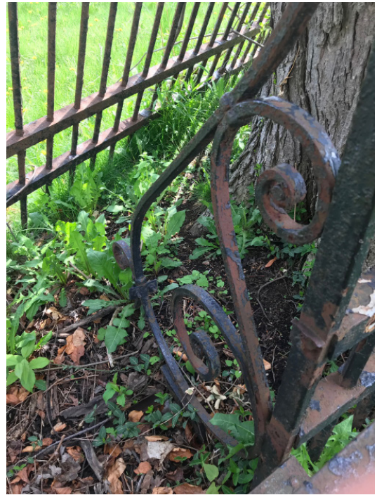
Existing condition of the iron fencing (ERA, 2018).
