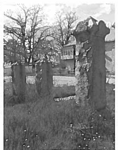
06 Existing condition of the west gate posts at the sidewalk entrance prior to the reinstatement of fencing, gates, lanterns and plaques (EPA, 2018)
