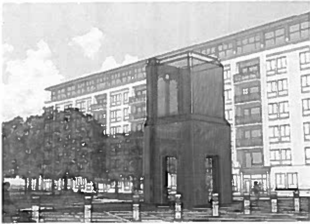
Commemorative Spire structure at termination of Moore street axis
