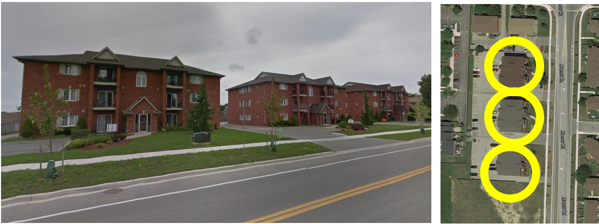
Figure 10: Manor Road Apartments
