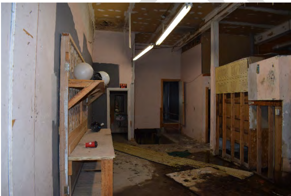
Plate 40: Looking north in garage door area of addition
