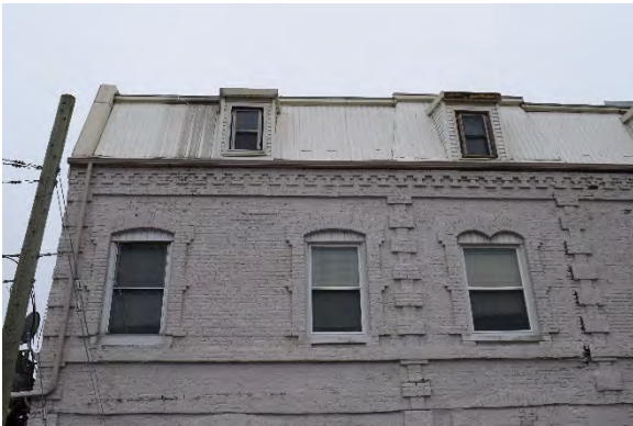
Plate 24: Details of visible sections of second storey windows, 248 Talbot Street looking west
