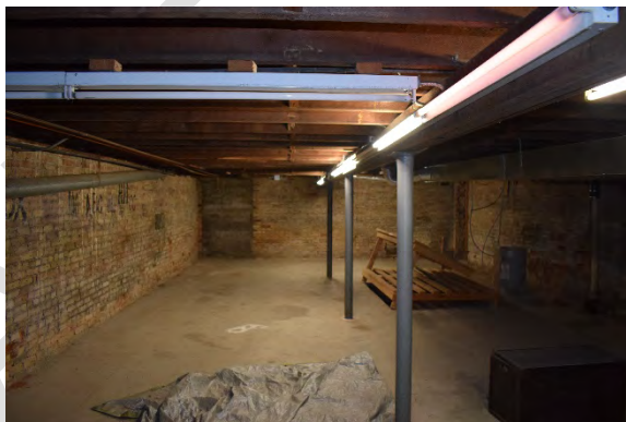
Plate 33: Basement of 246 Talbot Street, looking north
