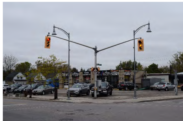
Plate 11: Looking northwest at intersection showing traffic lights
