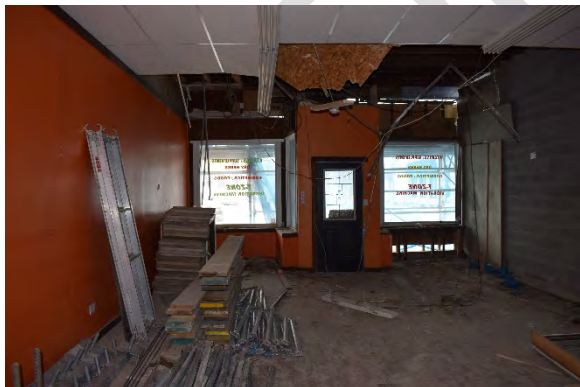
Plate 34: First storey of 248 Talbot Street, looking north
