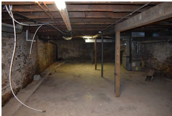
Plate 31: Basement of 244 Talbot Street, looking north
