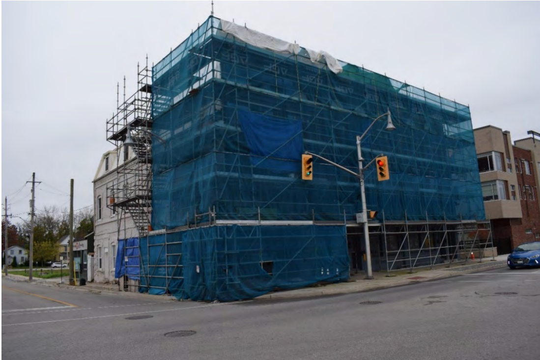
Plate 14: Scaffolding partially obscuring views, looking southwest
