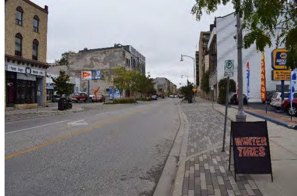
Plate 7: Looking east on Talbot Street showing commercial character
