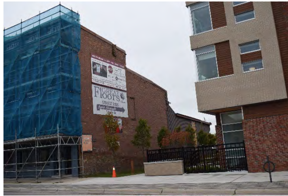
Plate 17: West elevation of 244 Talbot Street, looking southeast
