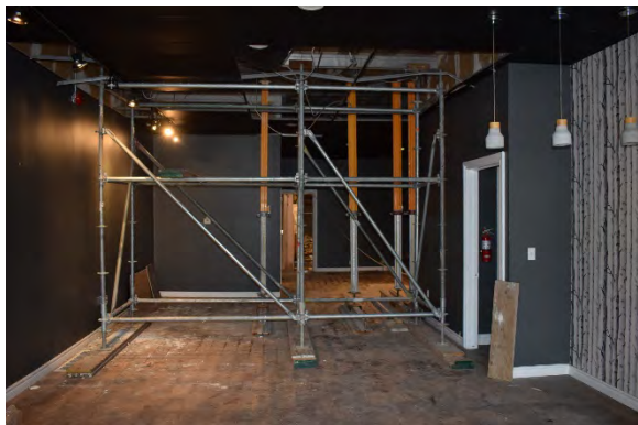
Plate 30: First storey of 244 Talbot Street, looking south
