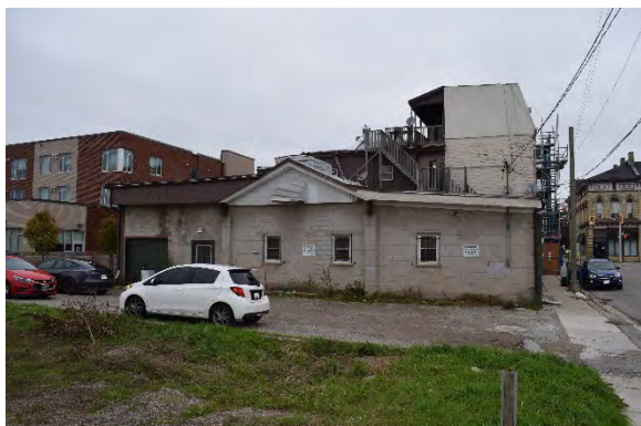
Plate 12: Gravel driveway, looking north towards 244, 246, and 248 Talbot Street
