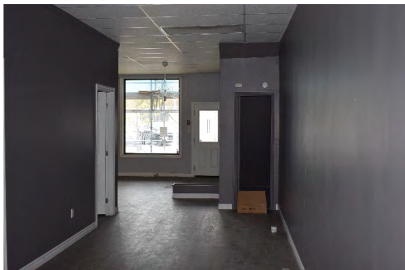
Plate 32: First storey of 246 Talbot Street, looking north
