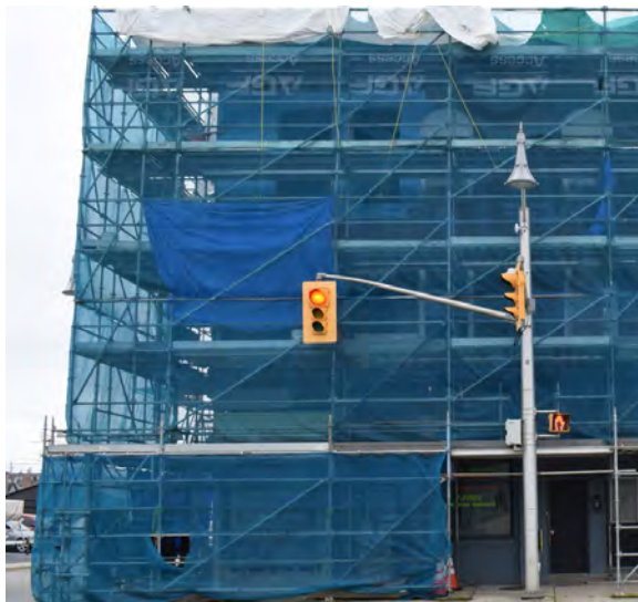
Plate 21: Front façade of 248 Talbot Street, looking south
