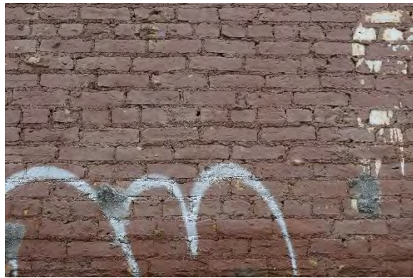
Plate 18: Brick bond of 244 Talbot Street, looking east
