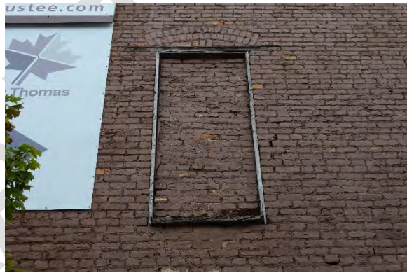
Plate 19: Blind window, 244 Talbot Street, looking east
