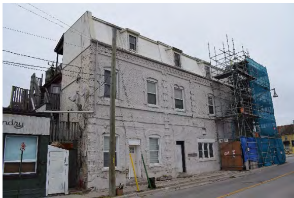
Plate 22: East elevation, 248 Talbot Street, looking northwest
