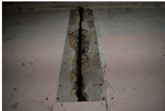
Plate 41: Wall gap, looking east
