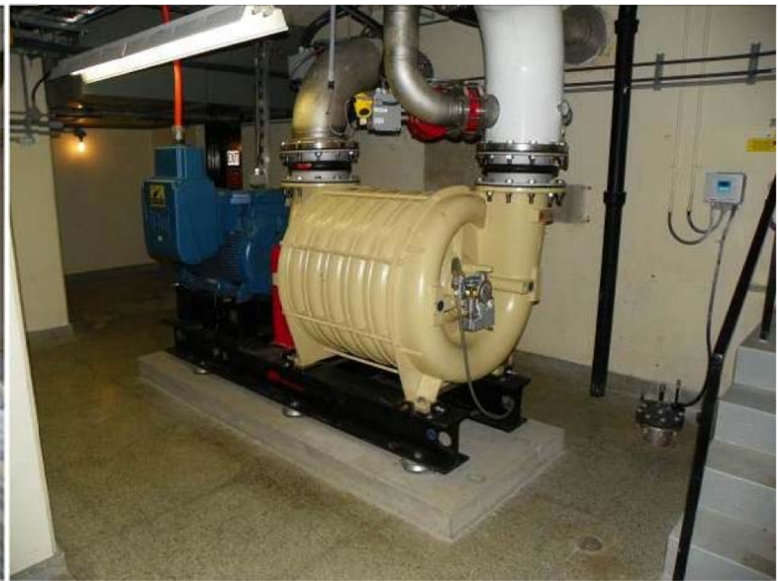
Filter 7: The air scour blower provides air to the filter during the air scour cycle of a filter backwash.
