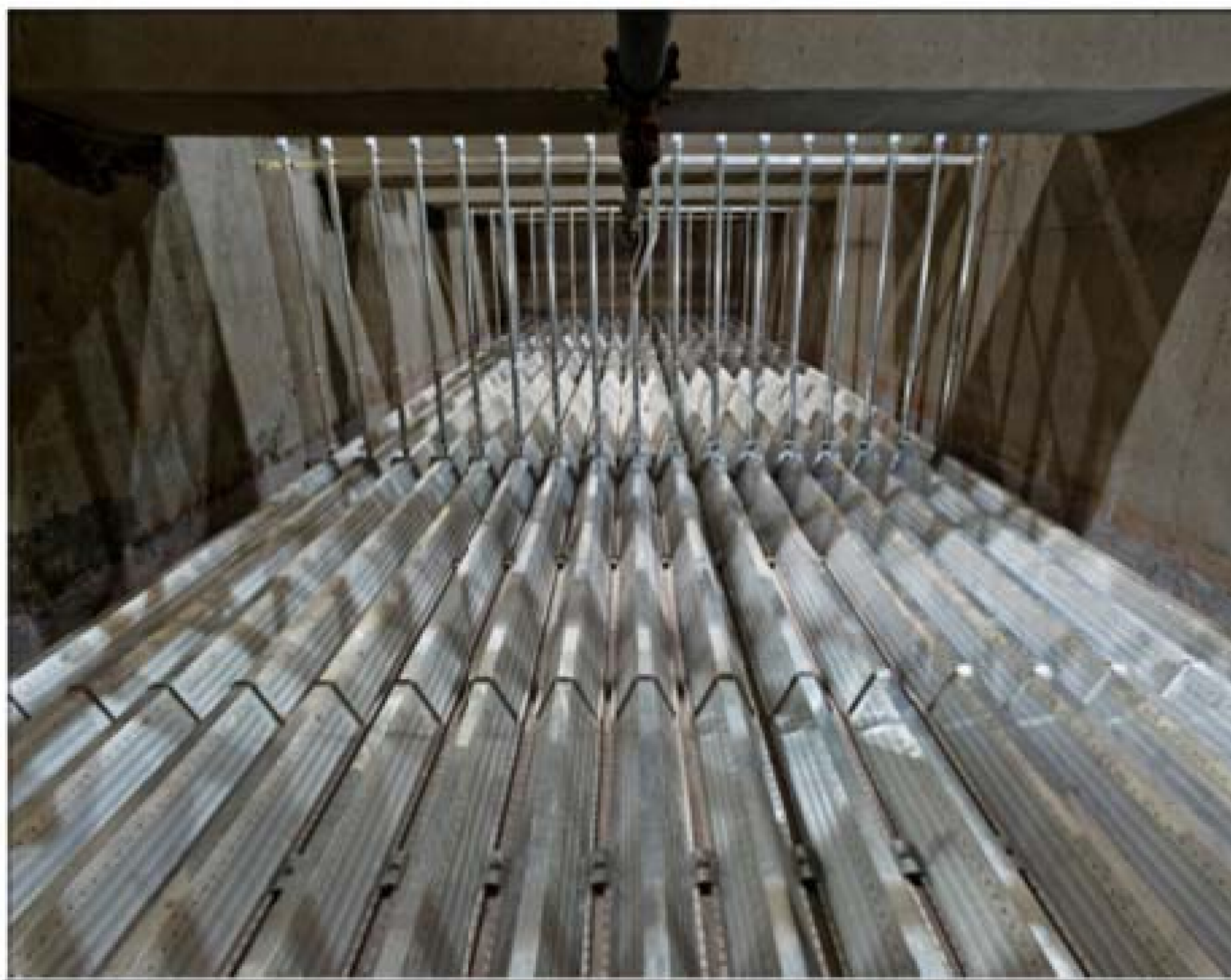
Figure 6: Completed installation of the new stainless steel underdrains and air scour piping in Filter #4.
