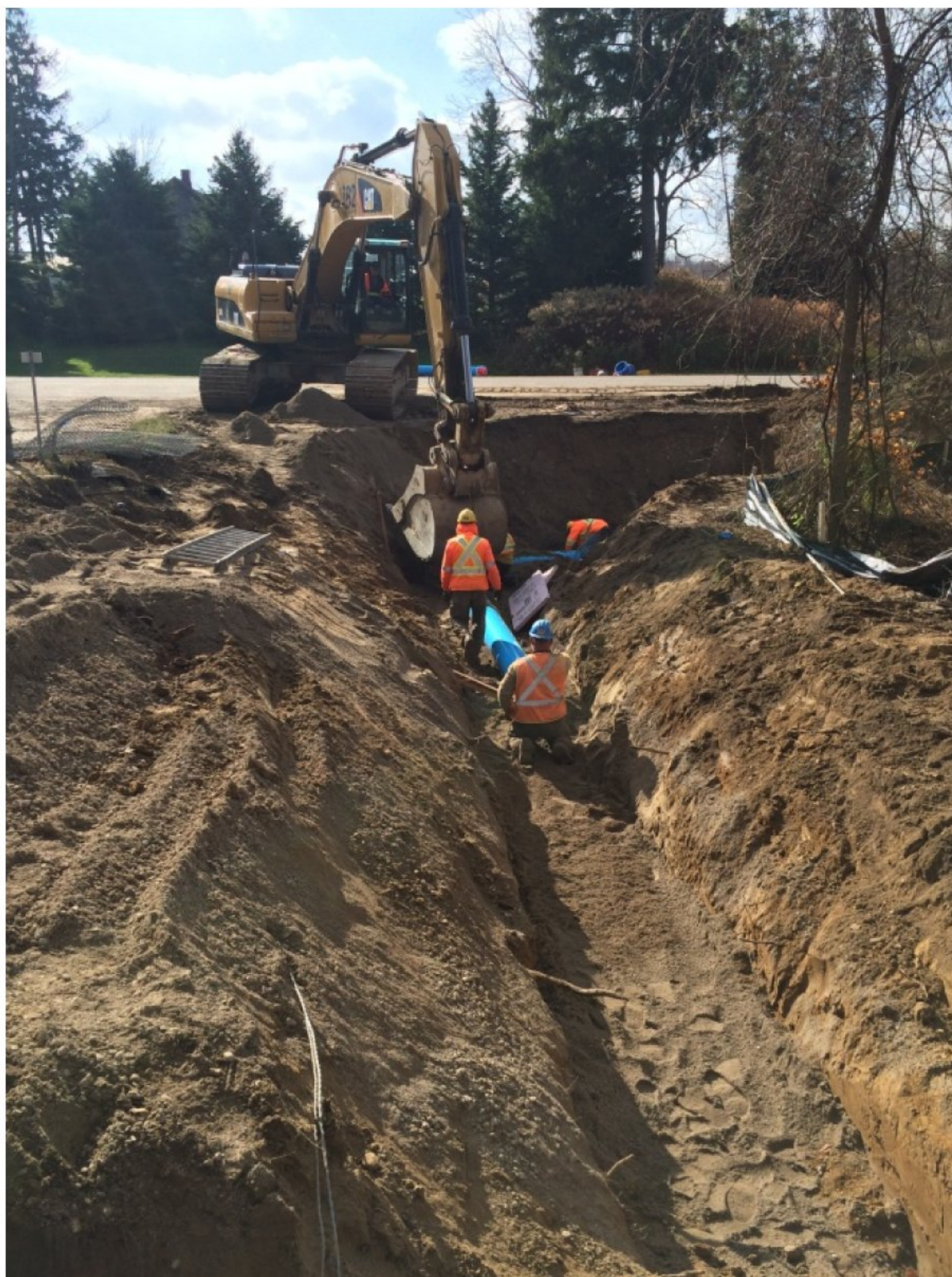
Figure 6: Installation of the new watermain.
