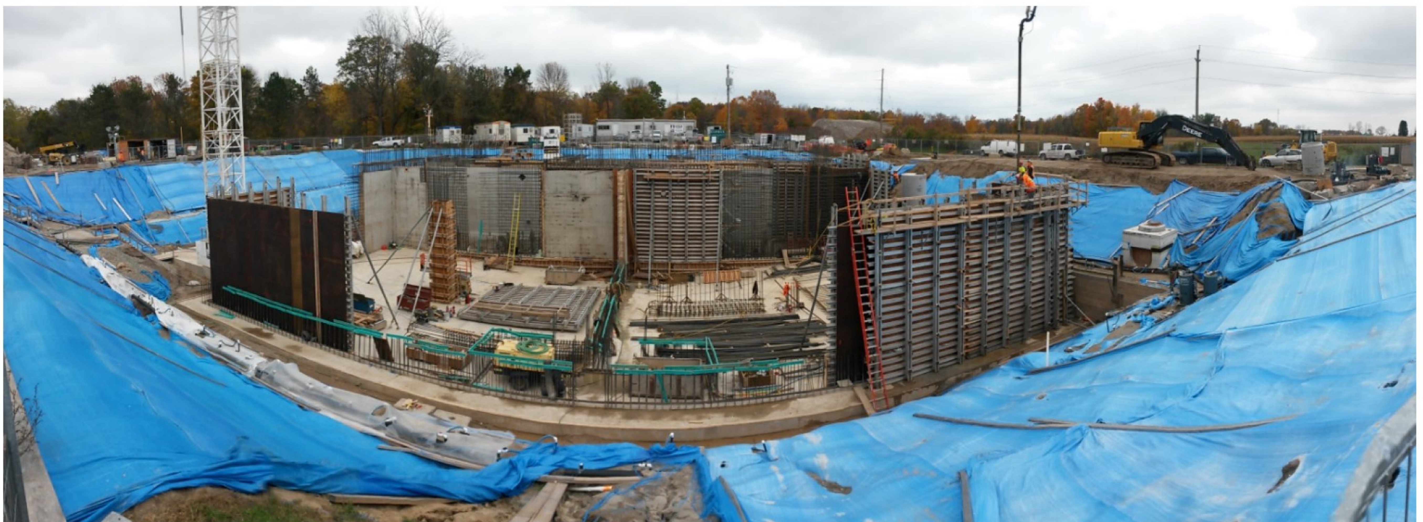
Figure 5: Setting up concrete forms for the walls.
