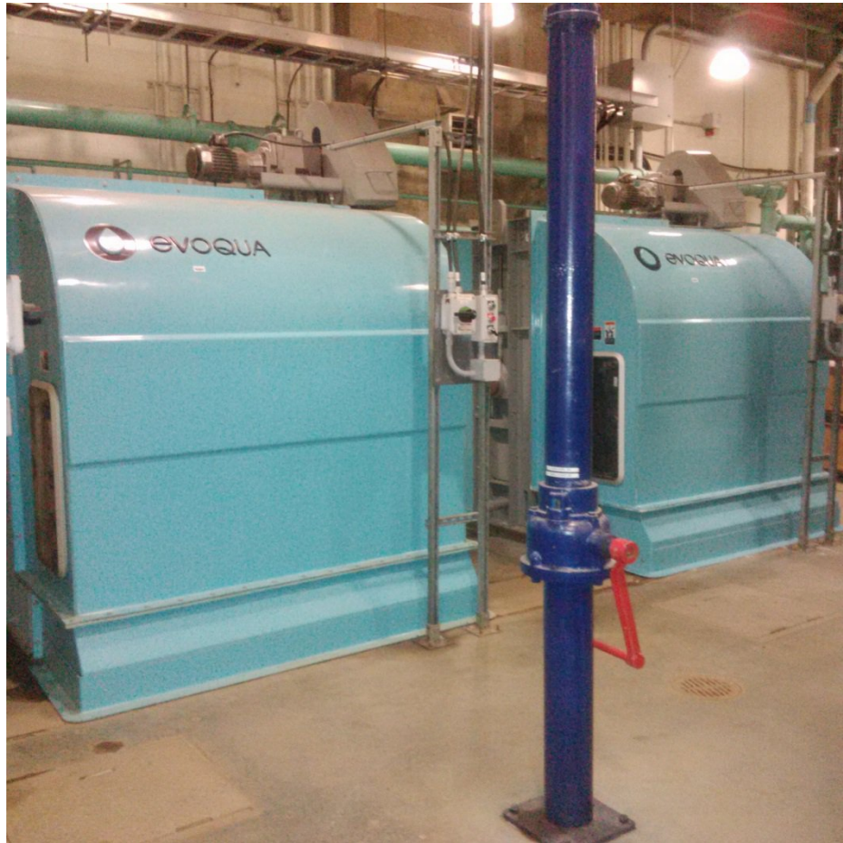
Figure 5: Two new travelling screens located in the low lift building.
