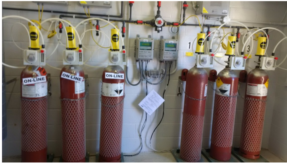
Figure 6: New 68 kg chlorine gas cylinders; chlorine gas is used for zebra mussel control.
