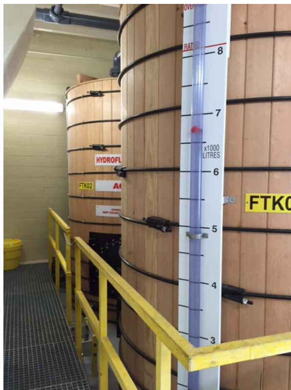
Figure 7: Two new wood stave bulk chemical storage tanks.
