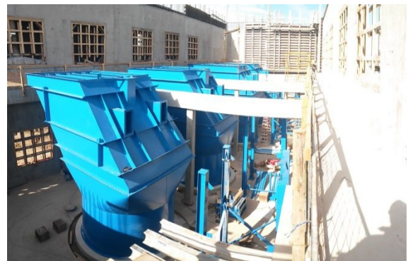
Figure 8b: April 15, 2015; Thickener units being installed.
