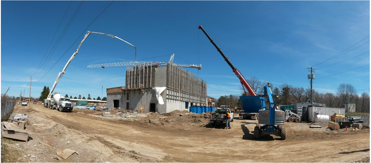
Figure 8c: April 15, 2015; Second floor concrete wall pours.
