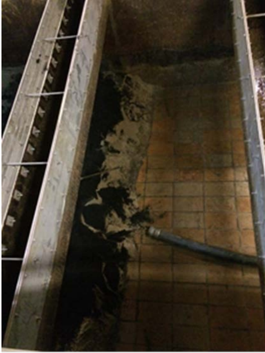
Figure 8a: Removal of the previously existing filter media (sand and anthracite), exposing the old clay tile underdrains.
