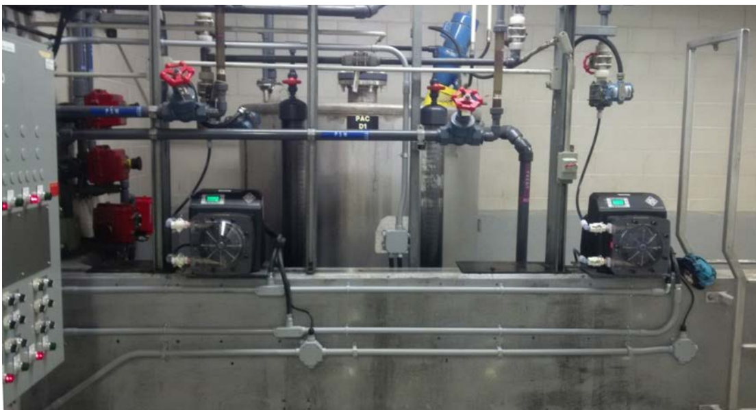
Figure 6: New carbon pumps
