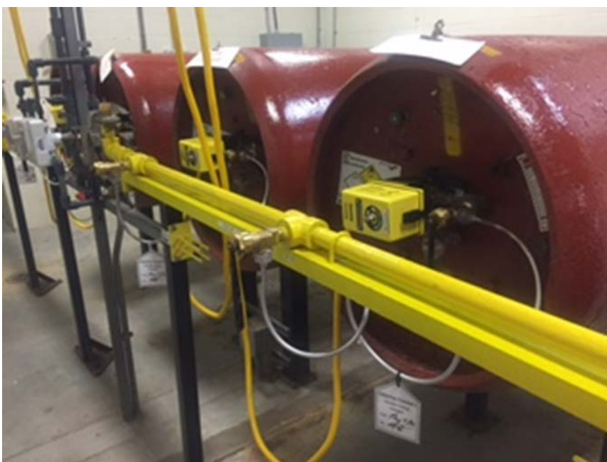
Figure 7: Chlorine tonners with emergency actuated valves
